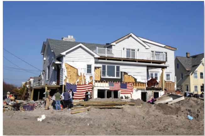
IMAGE 8-5 After Hurricane Sandy in 2012, volunteers help to rebuild homes destroyed in Far Rockaway, New York.
